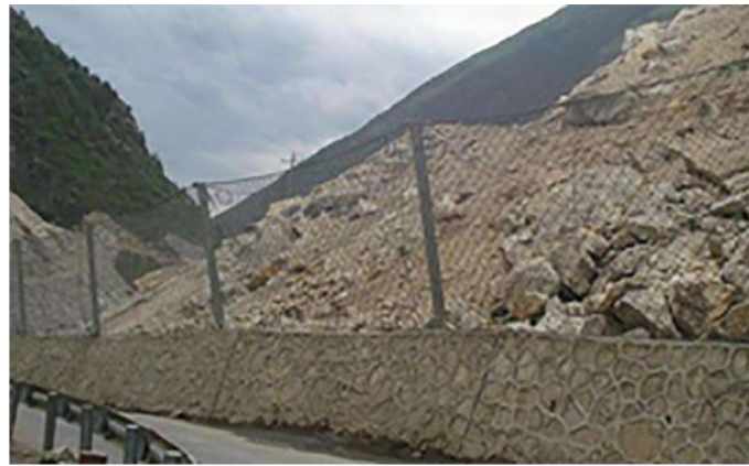
Fig. 2 Application of Passive Rockfall Barriers in Practical Engineering
